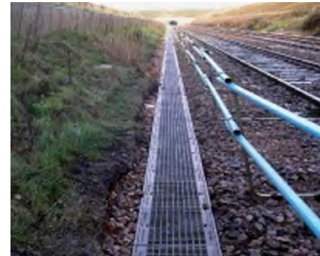
IMPROVED PERCOLATION ALONG RAILWAY LINE Severn Tunnel East, UK
