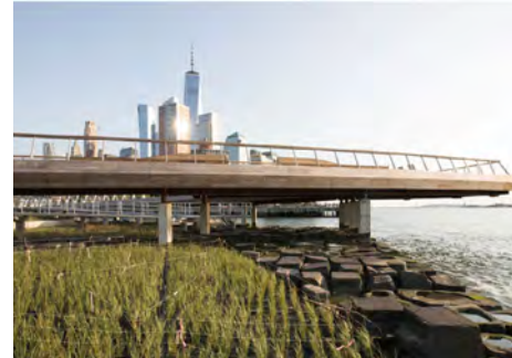
ELEVATED BOARDWALK INTEGRATED WITH NATURE- BASED COASTAL PROTECTIONS Pier 26, Hudson River Park, New York City
