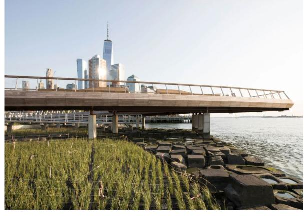
ELEVATED BOARDWALK INTEGRATED WITH NATURE BASED COASTAL PROTECTIONS
